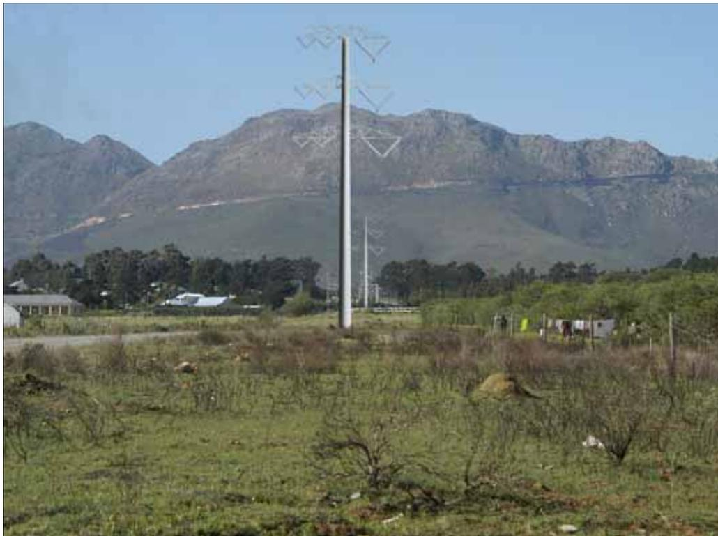
**Photograph 2.1:** Monopole structure which can be used in areas where there are space constraints
